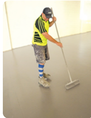
Application of MasterTop 1080
